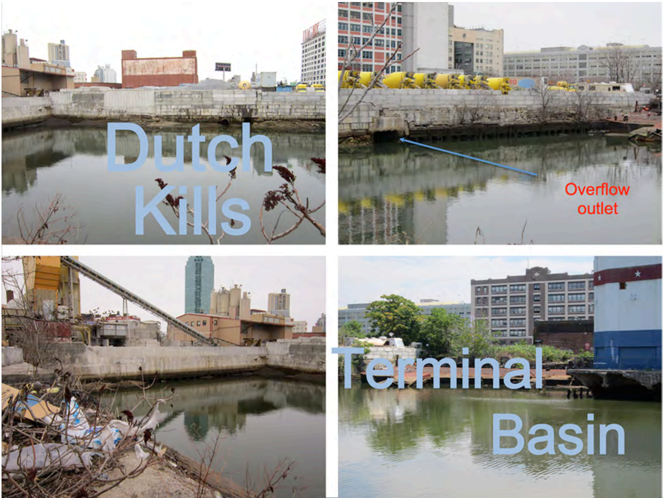
Fig. 4. Dutch Kills Terminal Basin: a human engineered dead end. Arrow points to "CSO" (see text) - photos by Sarah Durand
